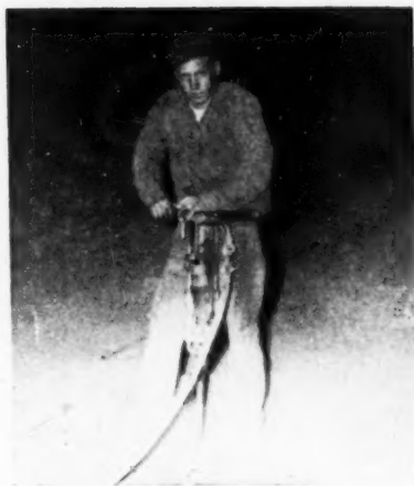
Driller Bill Courson operates a Gardner-Denver S-55 Sinker putting down holes in waste just above the orebody. Bill lamps the cuttings frequently and, at about eight feet in this hole, entered the ore and stopped drilling.
